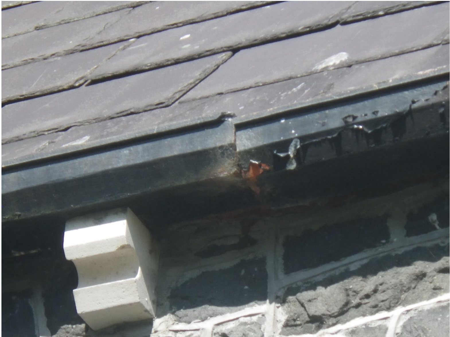
Broken gutter
