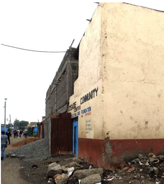
.....and during the extension
