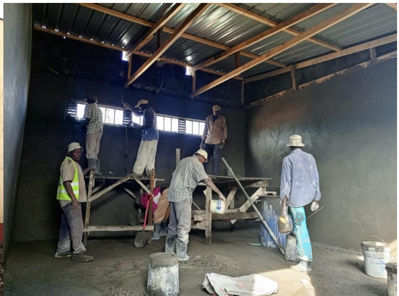
one of the new classrooms being built
