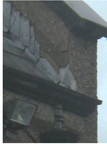
St John's flashing
