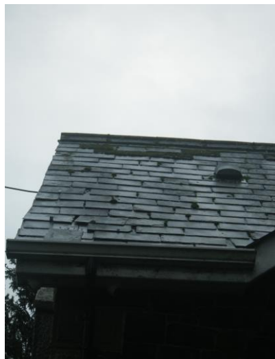
Slipped and dislodged slates to front slopes.
