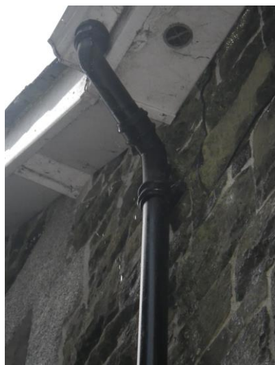
Leaking rainwater goods
